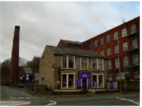
6 Spottland Bridge Mill
