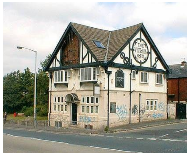
Former Victoria Hotel, Spotland Road, prior to cladding of gables
