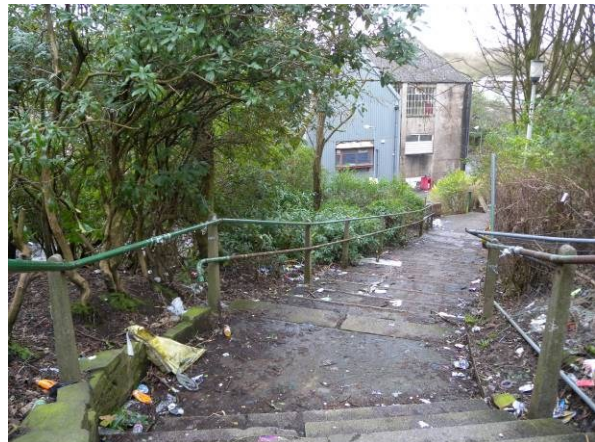
Unsecured steps access
