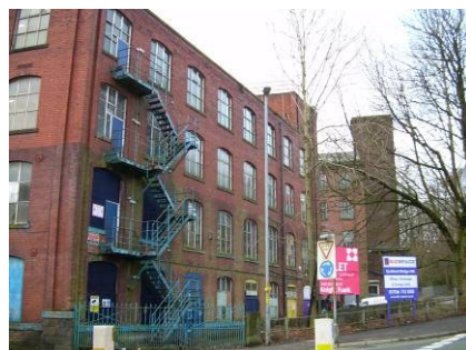
Four storey mill building
