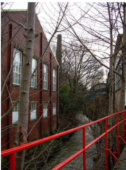
View to Spotland New Mill, River bed
