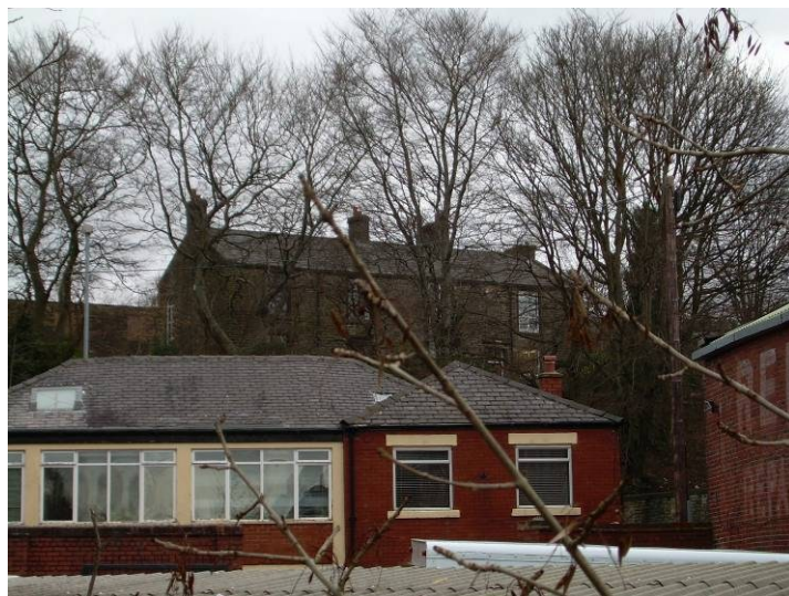
Roofscape, view from the river at Spotland Bridge
