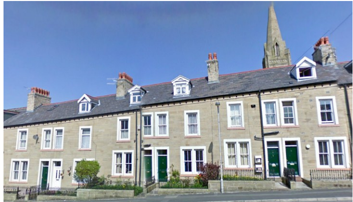
Restored terraces in Meadow Bank Road Nelson, Lancashire
