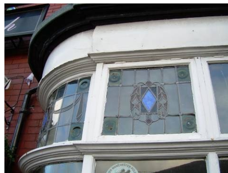
Original window detail
