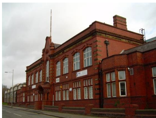
Former Tramway Depot, Mellor Street
