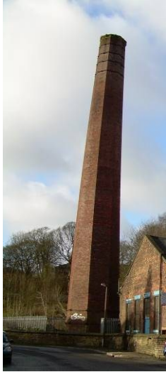
Spotland Bridge New Mill chimney
