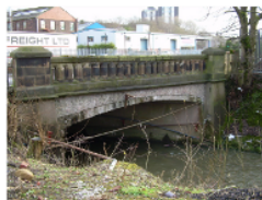
Listed concrete bridges 9
