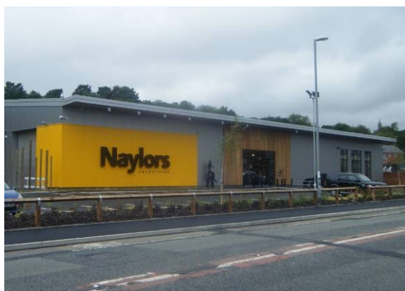
Naylor's commercial unit, Mellor Street
