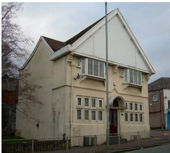
Former Victoria Hotel, Spotland Road, in present condition.
