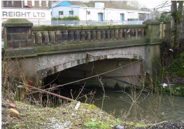
Mellor Street Bridge, View from Naylors' site
