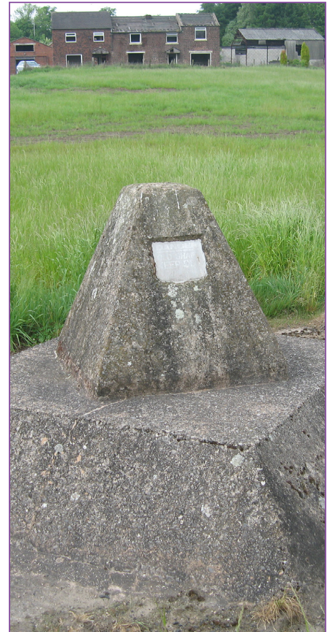
Capped mineshaft at Site 1
