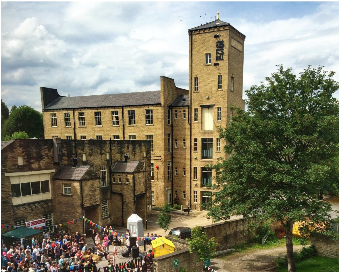
2 Sunny Bank Mills, Farsley, Leeds
