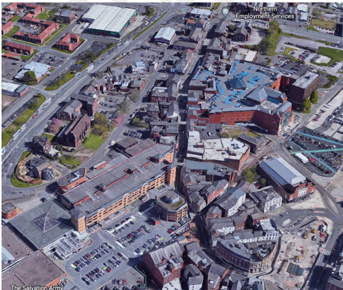
Below—Google Earth Aerial 3D Image of Yorkshire Street — Google Earth
