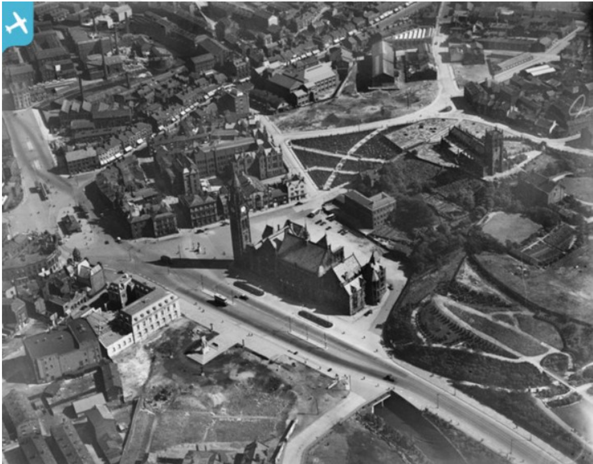
Copy of Aerial photograph from Historic England—Britain From Above Collection— Town Hall Square, Rochdale, 1926
