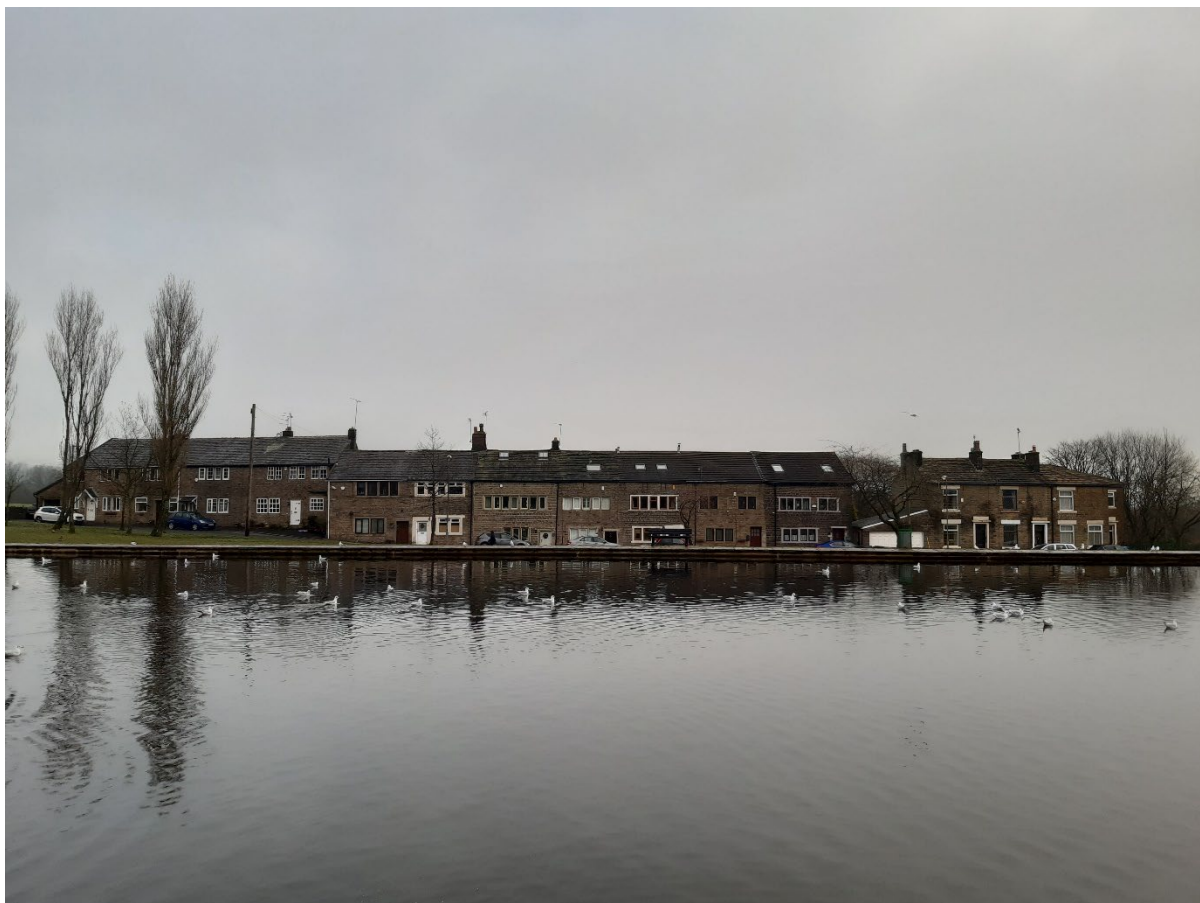
Figure 22 - Weavers Cottages at Polly Green, Syke Road
