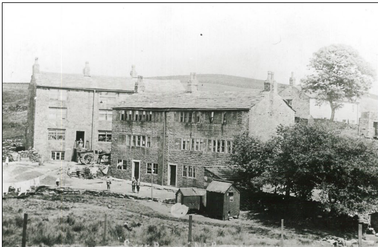
Figure 41 - Demolished weavers' cottages at Syke Bottom
