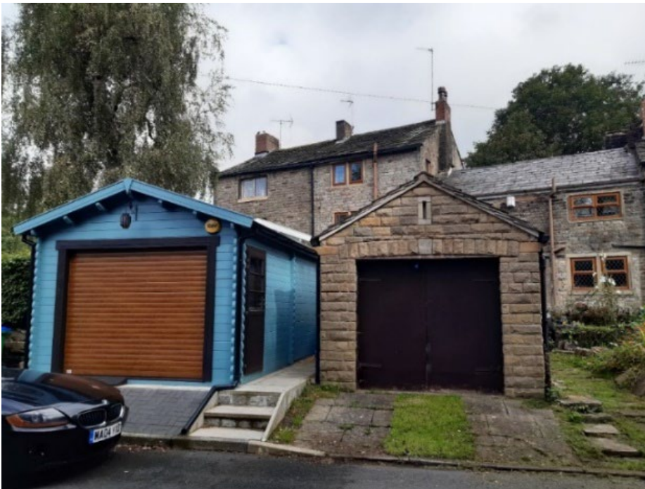
Figure 56 - Incongruous outbuildings on Syke Lane
