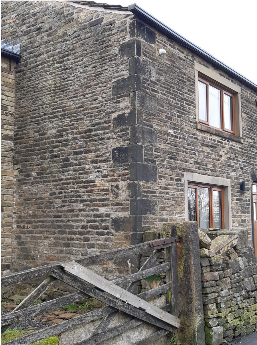
Figure 18 - stone quoins on historic buildings
