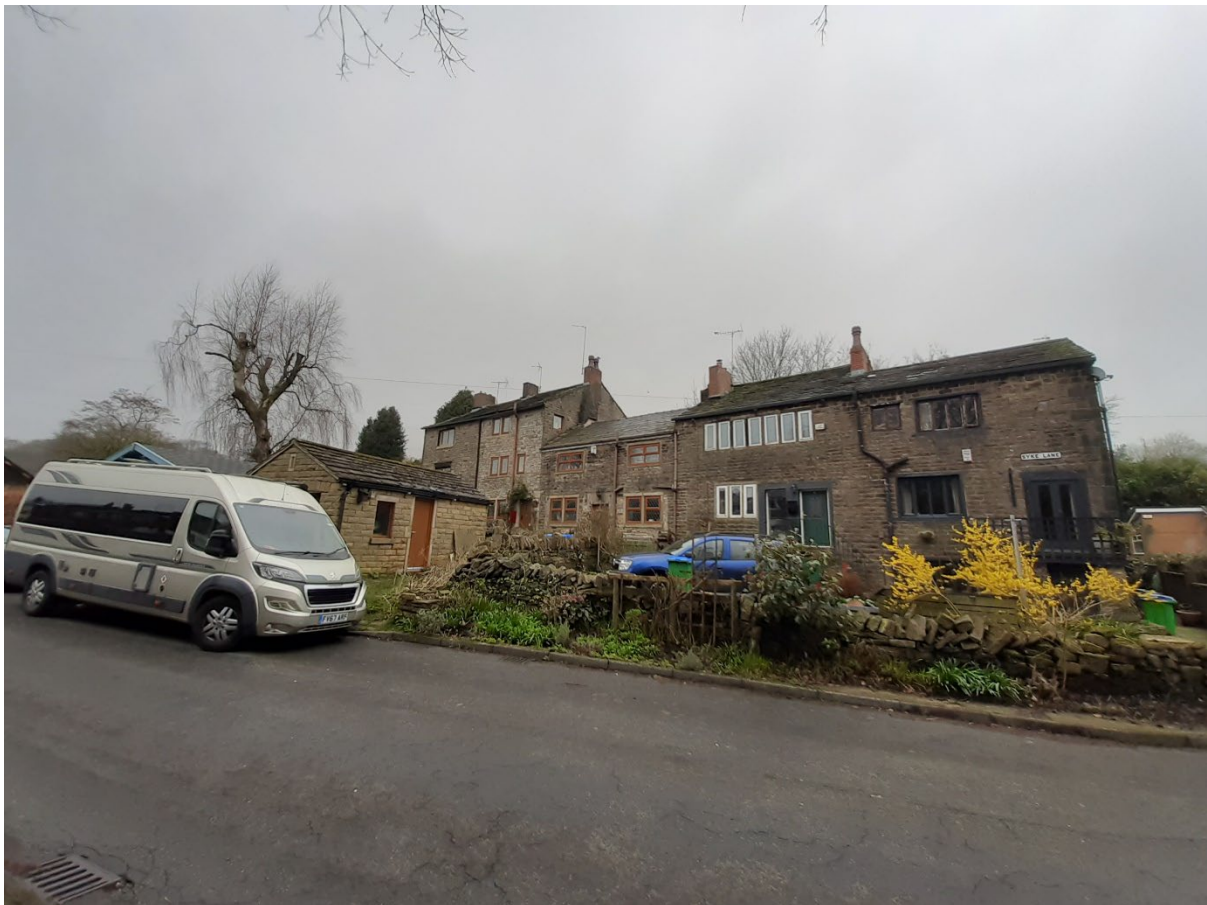
Figure 28 - Houses on Syke Lane
