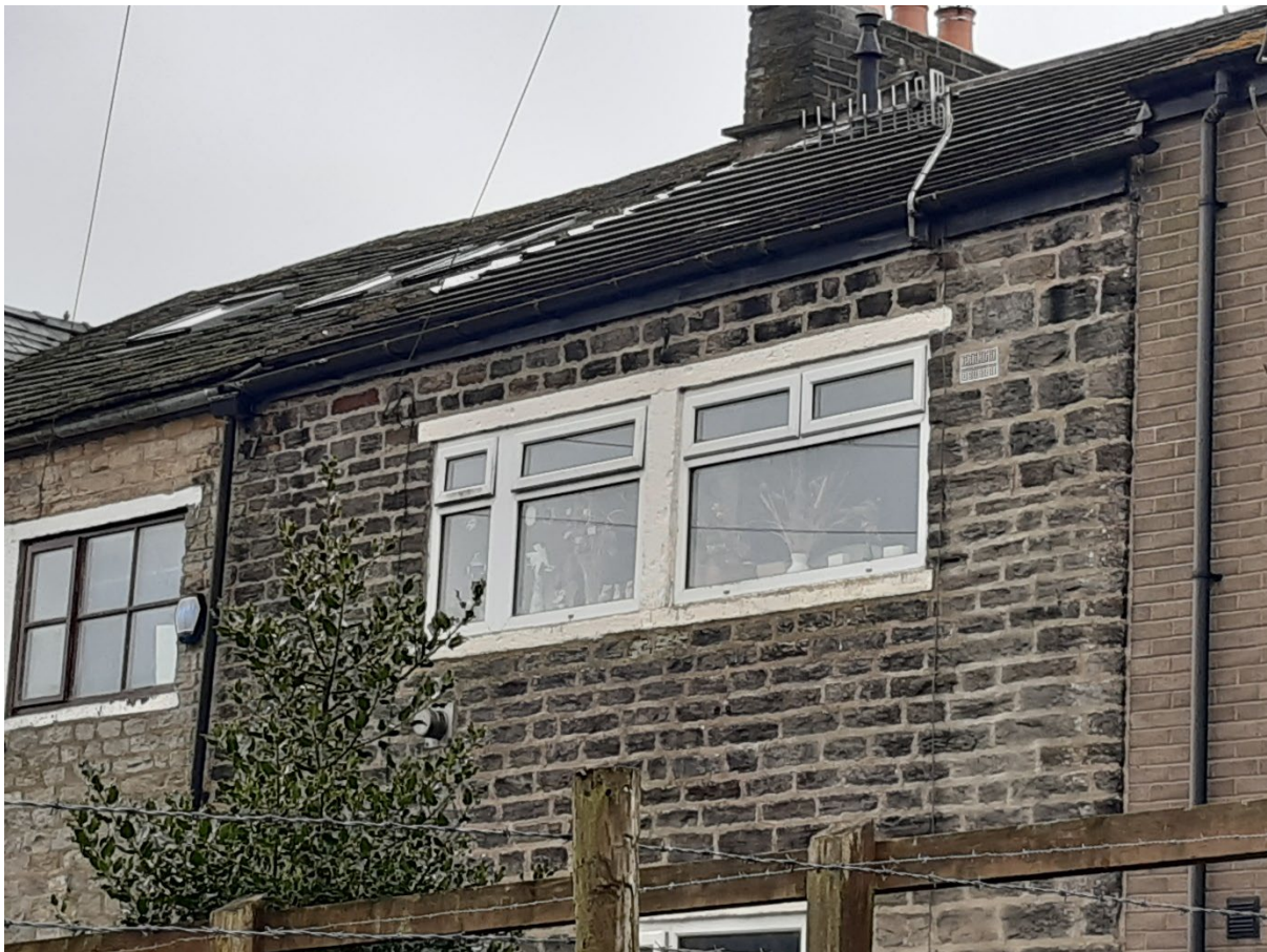
Figure 54 - original stone mullions removed and uPVC windows installed
