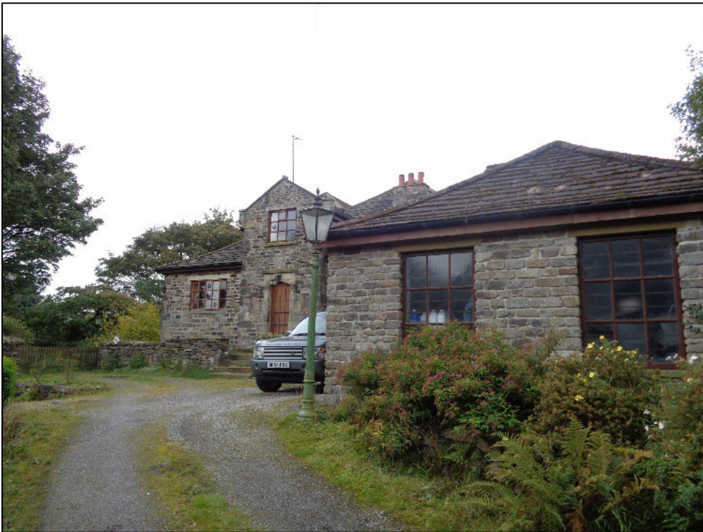
Figure 4 - Dwelling on the site of the former Cordwainers Arms
