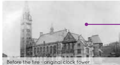
Before the fire - original clock tower
