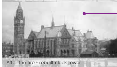
After the fire - rebuilt clock tower
